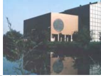
Baltimore's waste to energy plant – BRESCO – serves Baltimore's core/Downtown
